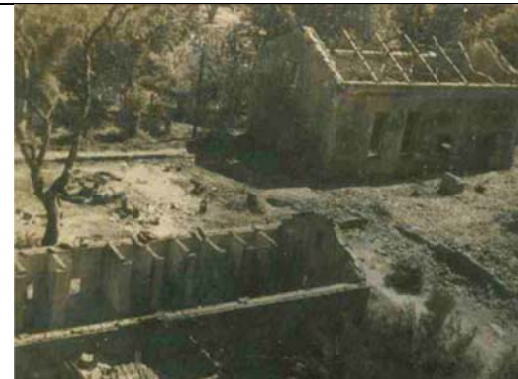
廁所、軍器庫毀損
